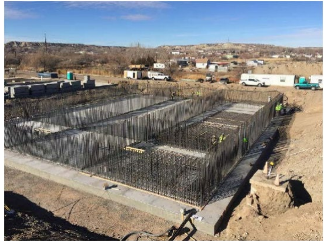
The Town of Bloomfield CWSRF 103 WWTP Construction
